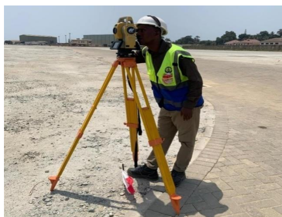
Establishing the corners of each parcel with Topcon Total Station
