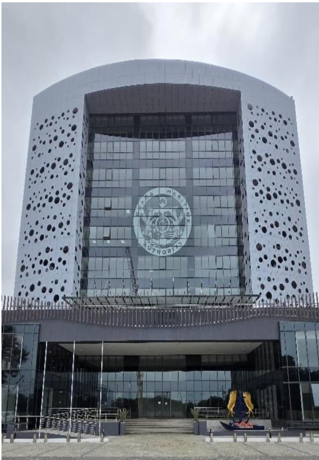
Head Office Building - Accra
