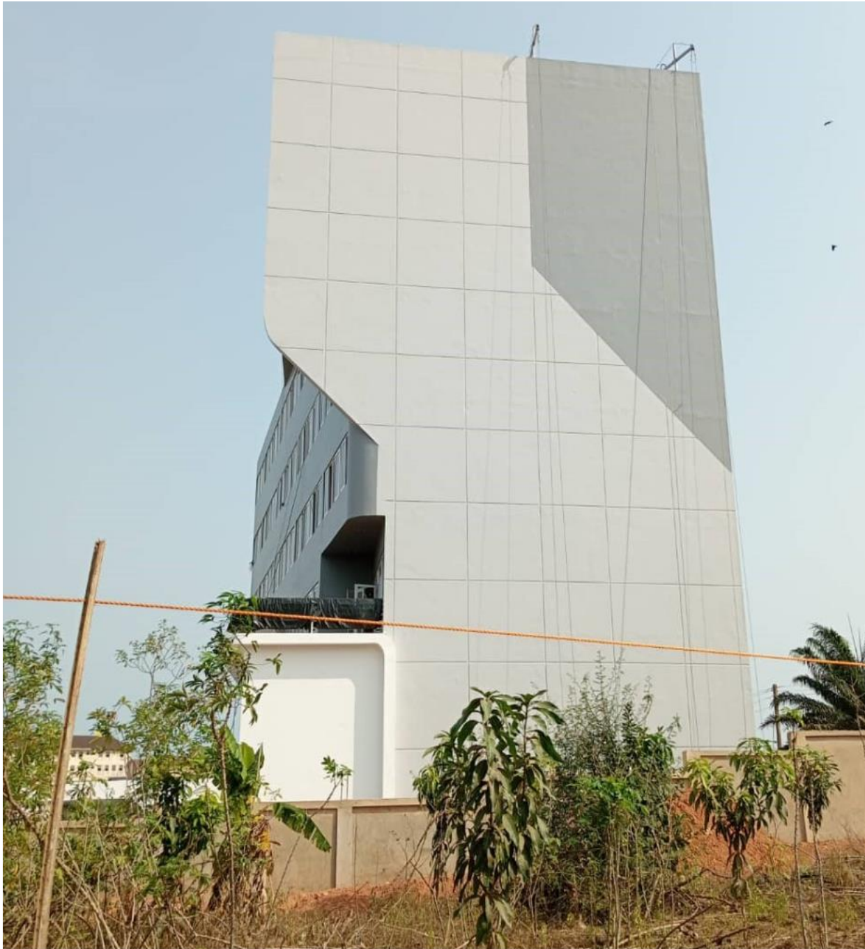
Takoradi Office Building
